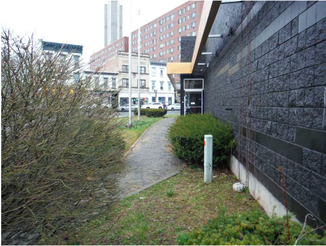
Photograph #17 – Overview of subject Property on April 4, 2024.
