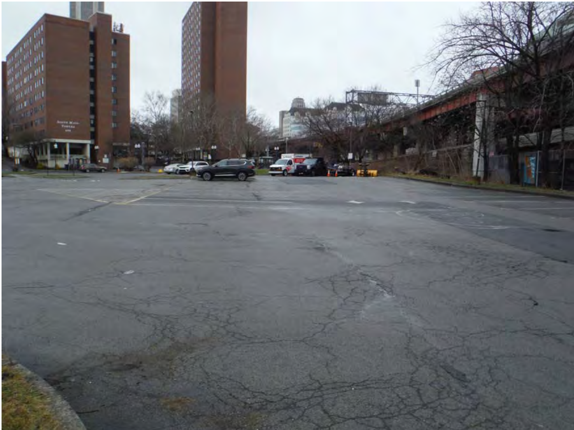
Photograph #16 – Overview of subject Property on April 4, 2024.
