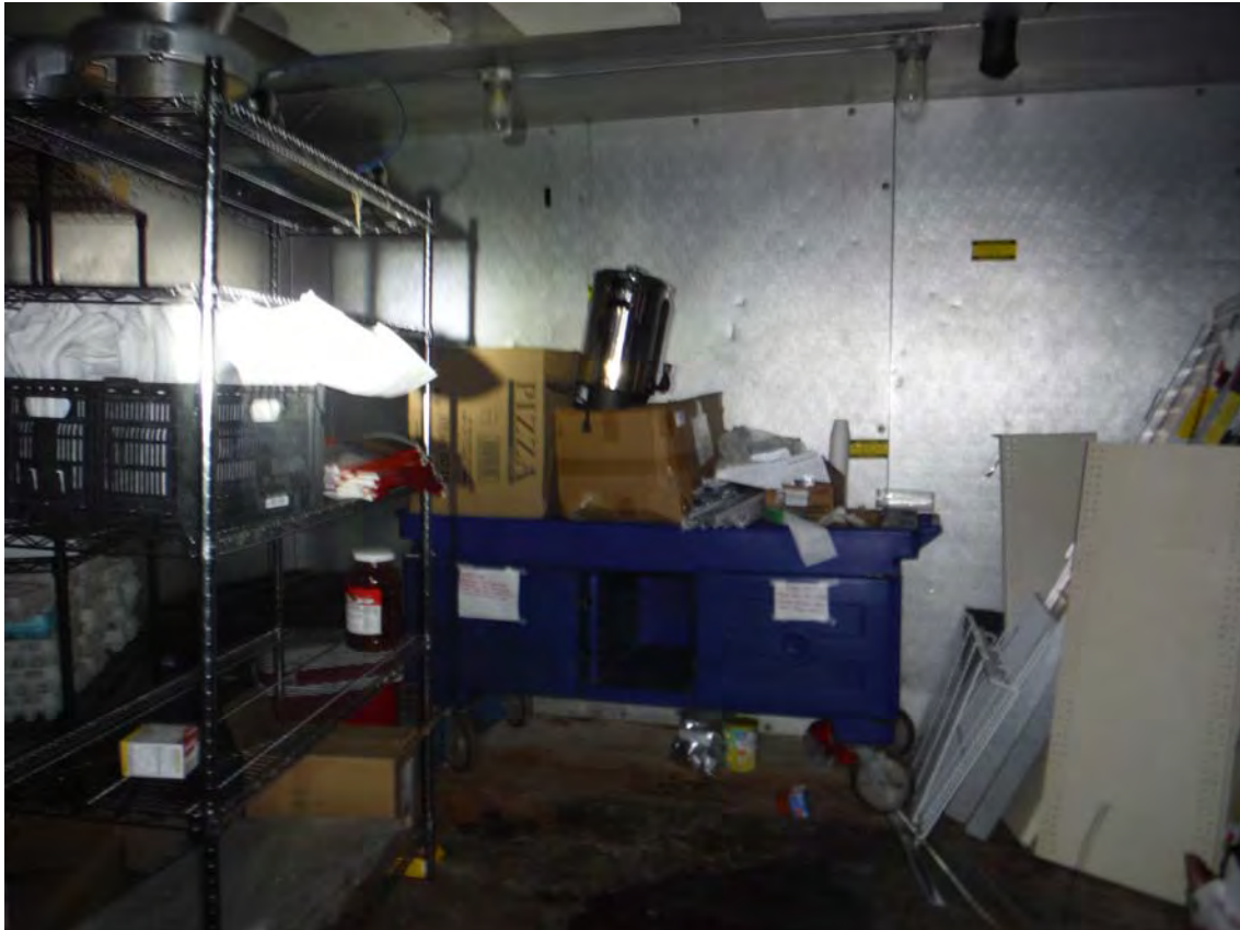
Photograph #13 – Overview of subject Property building on April 4, 2024.
