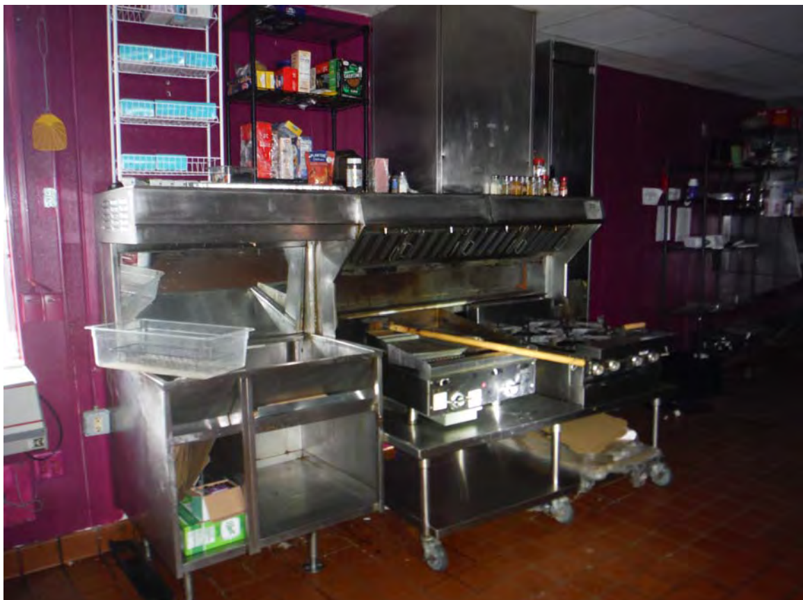
Photograph #4 – Overview of subject Property building on April 4, 2024.
