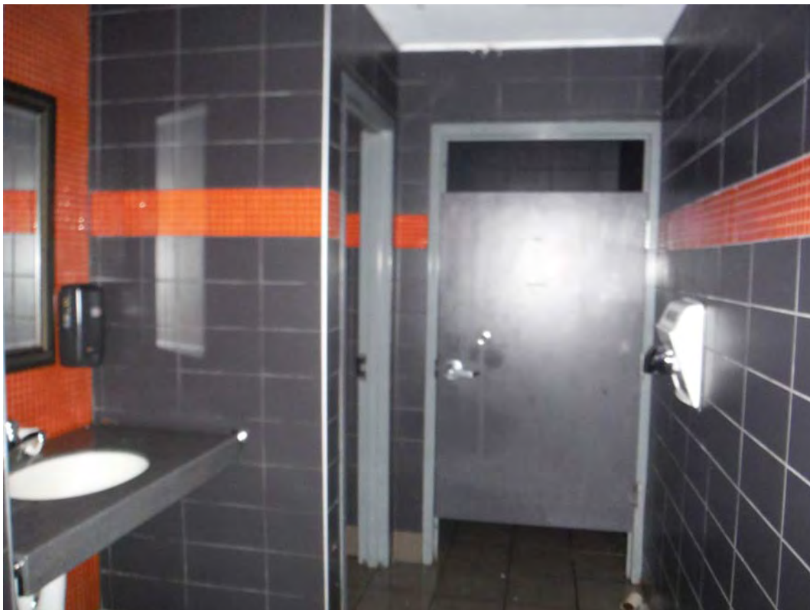
Photograph #10 – Overview of subject Property building on April 4, 2024.
