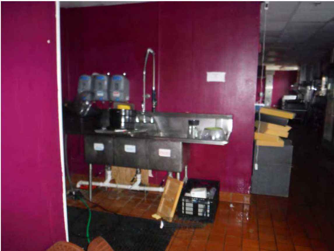
Photograph #8 – Overview of subject Property building on April 4, 2024.
