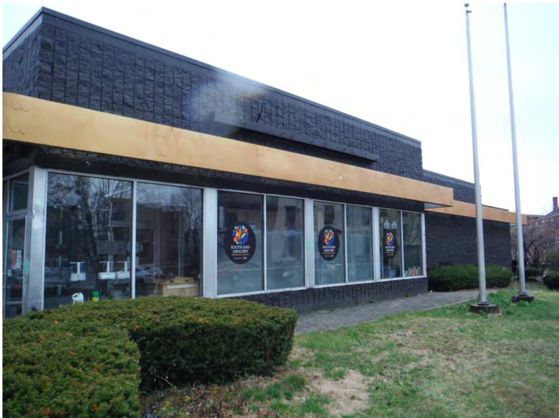
Photograph #2 – Overview of subject Property building on April 4, 2024.
