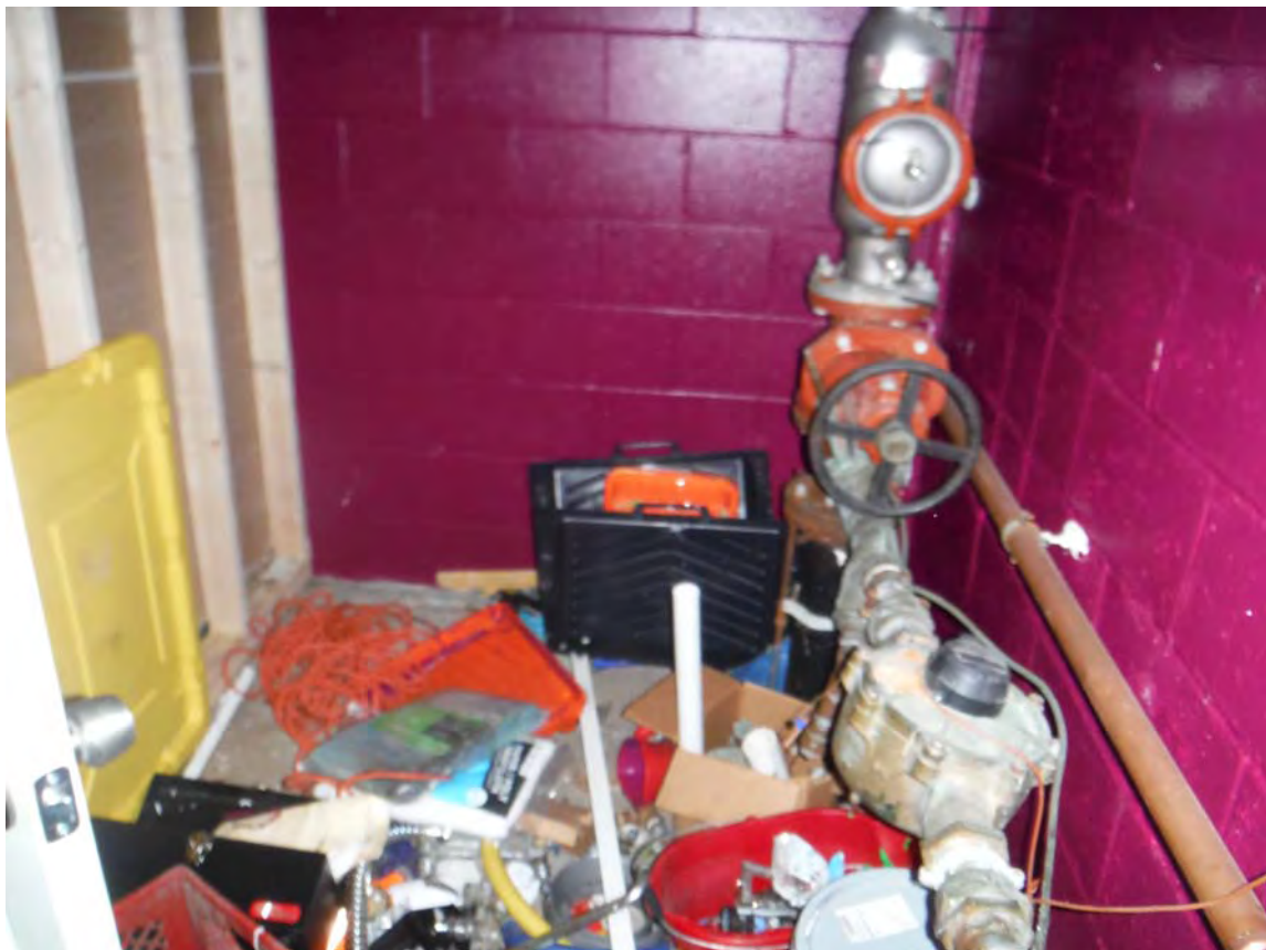
Photograph #12 – Overview of subject Property building on April 4, 2024.
