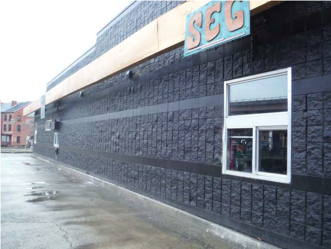
Photograph #15 – Overview of subject Property on April 4, 2024.
