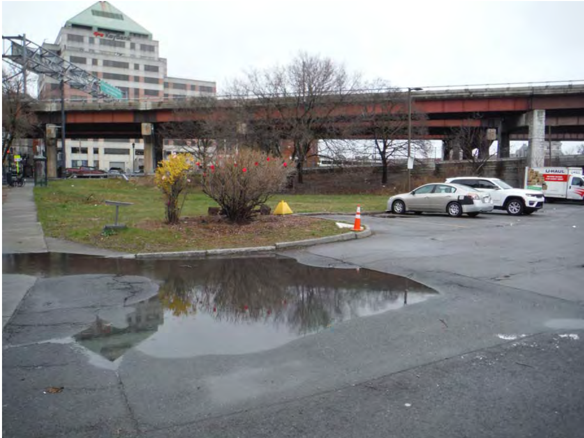
Photograph #19 – Overview of subject Property on April 4, 2024.
