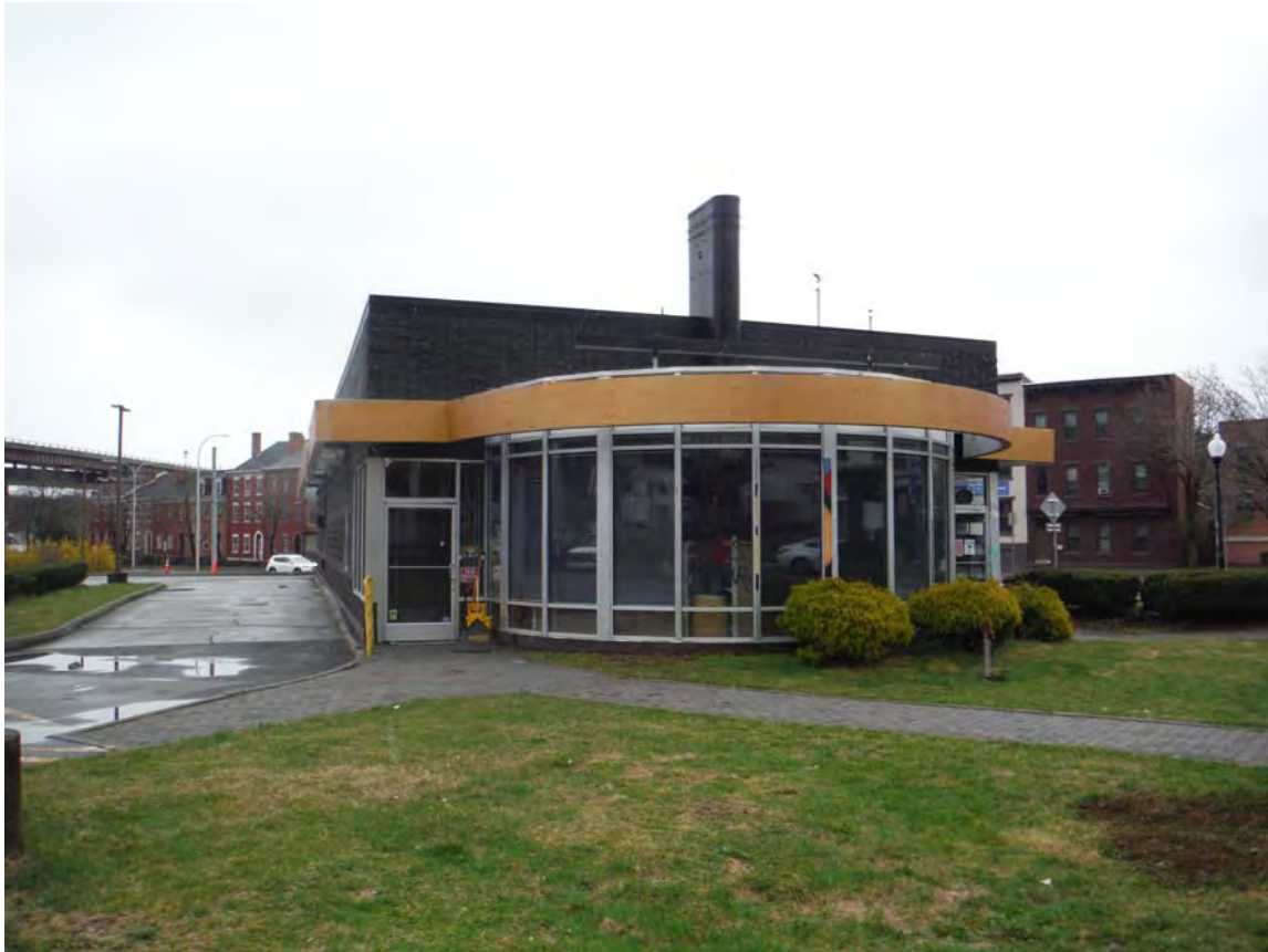
Photograph #1 – Overview of subject Property building on April 4, 2024.
