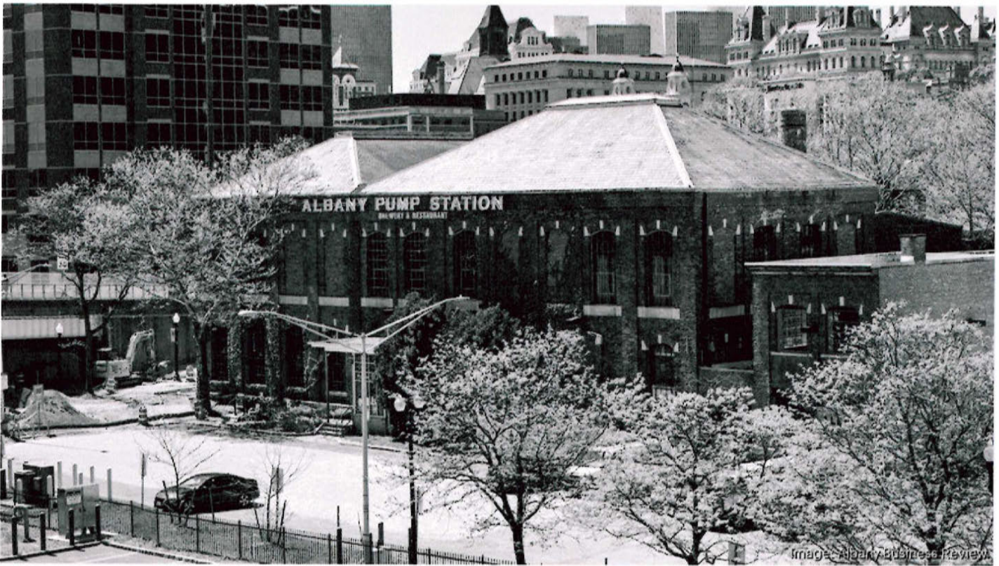
The Albany Pump Station building, shown here in 2022.
