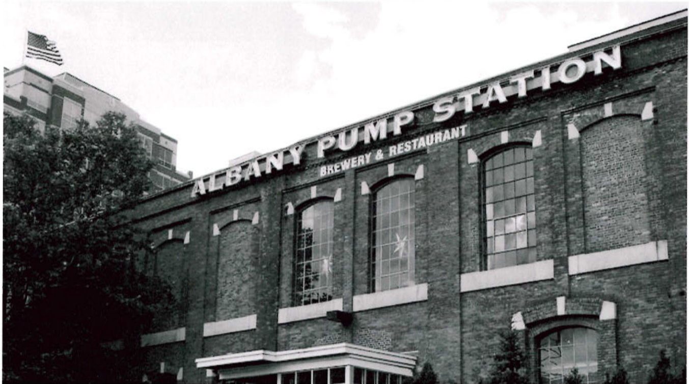
Albany Pump Station at 19 Quackenbush Square.
